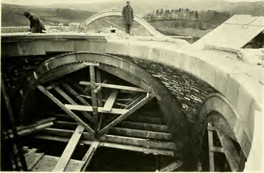
THE DOME IN CONSTRUCTION
